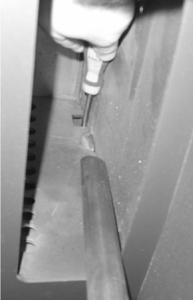
Figure 7: Removing ash from left hand landing cavity.
